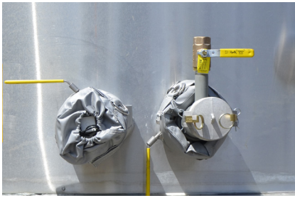
Dual insulated and heated valves
